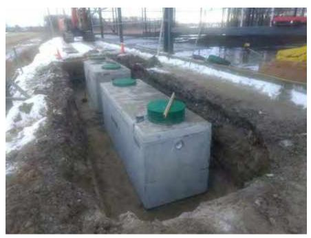
Figure 2.13 Installation of Bionest System
