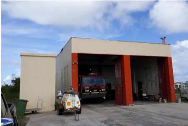
Barbuda Codrington Airport fire station hangar
