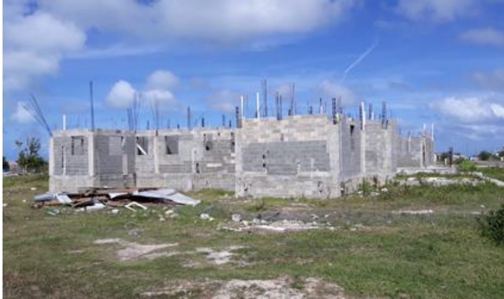
Barbuda Justice Center construction site
