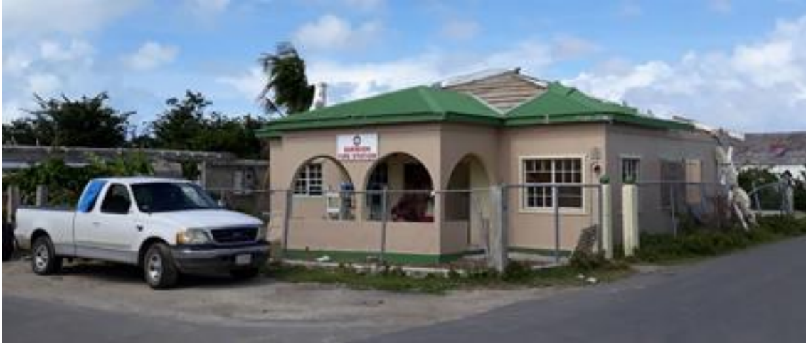
Codrington fire station
