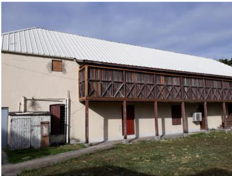
Clearvue – Male 2 storey ward, showing industrial sheet metal roof
