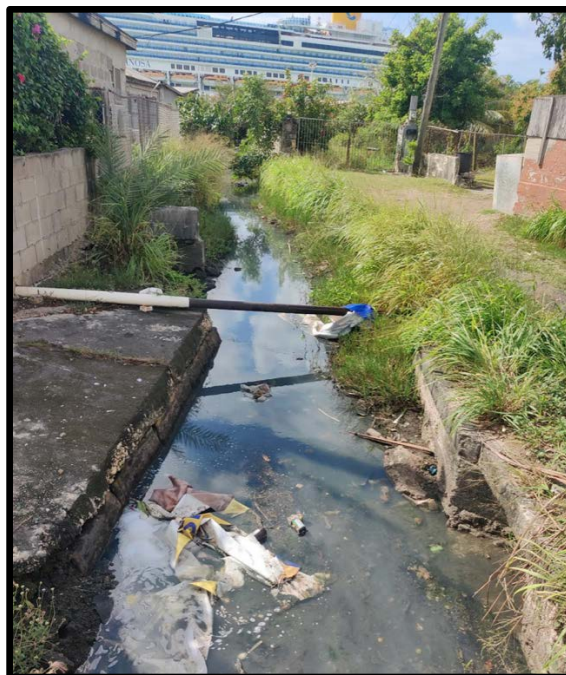
Figure 30: Open Drain 3 to the West of Barnes Funeral Home and North of Project Site
