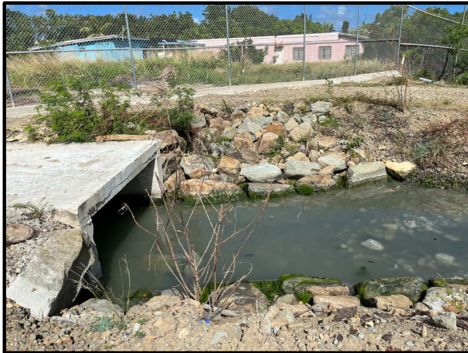
Figure 12: Concrete covering for formed waterway on project site
