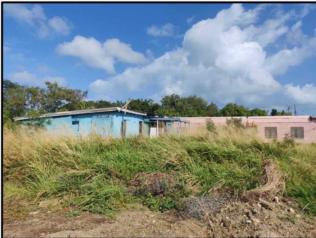
Figure 14: Current site conditions of proposed wastewater treatment plant location
