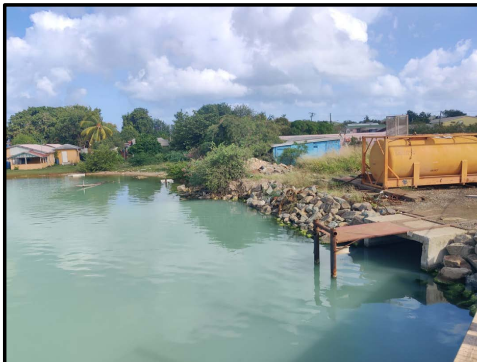
Figure 13: Continuation of concrete covering outlining discharge area from waterway on site
