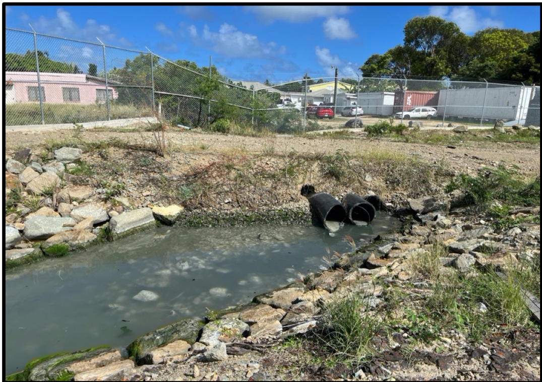
Figure 11: Community Drain within project site which is disposed into St. John's Harbour
