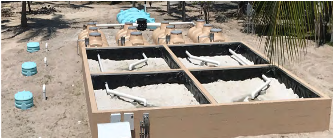
Figure 5.9.1. A Fujiclean forced-air wastewater treatment system with sand filter
